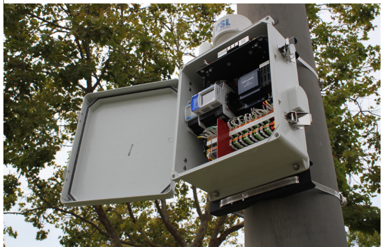
Figure 2: A \mu PMU installed on a utility electric distribution pole. The device consists of a high resolution power quality monitor and a GPS antenna (mounted on top of the box in this installation).
